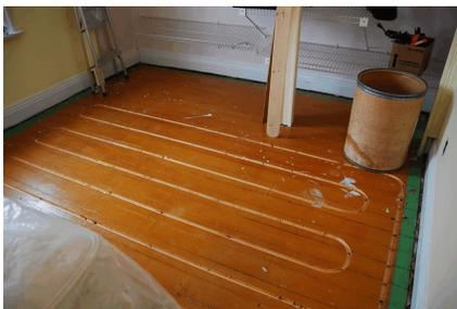
**Floor cut for heating pipe**
